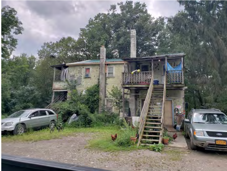
VIEW OF THE STRUCTURE FROM THE FRONT
