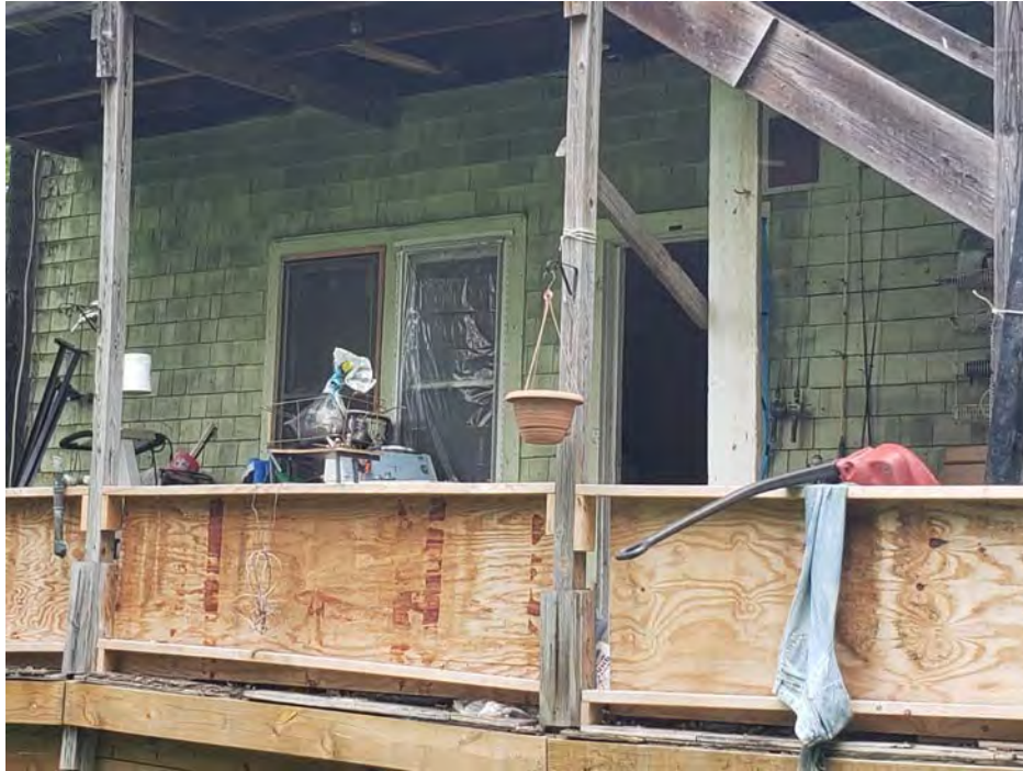
VIEW OF DOOR OPENING
