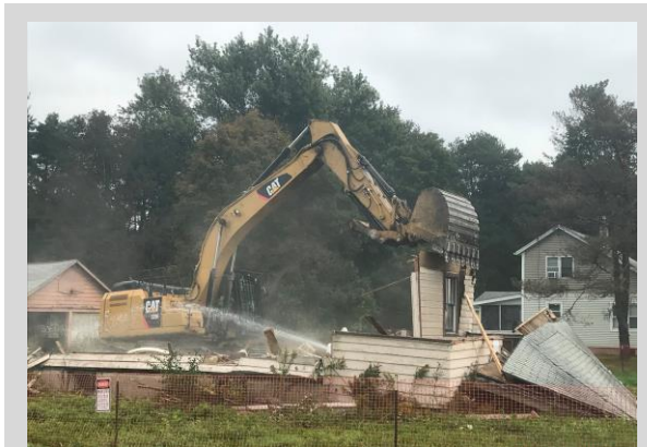
2977 NYS Route 26, Town of Maine
